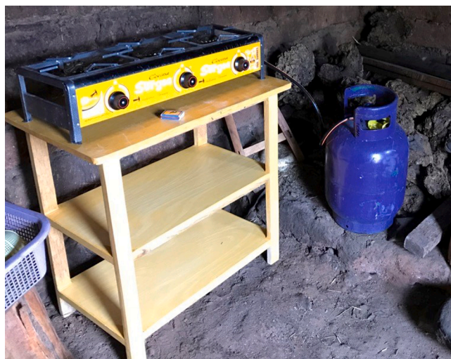
Fig. 1. Three-burner LPG stove with table and LPG cylinder, as installed in the kitchens of participants in the intervention group of an LPG cleaner-cooking trial in Puno, Peru.
